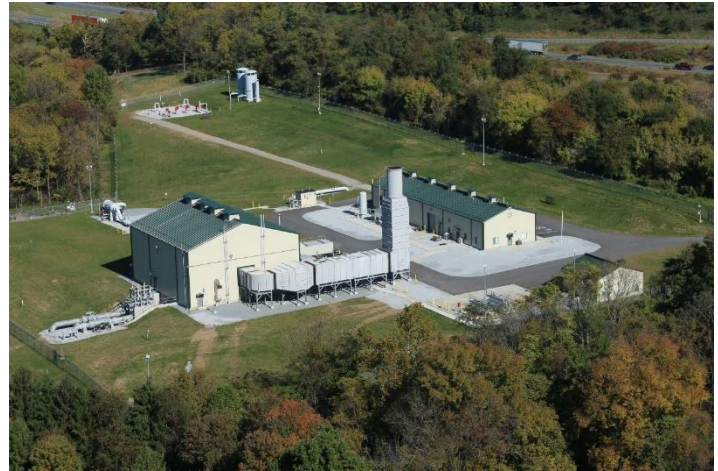
The EGTS Meyersville Compressor Station in Maryland.
